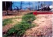
Sewage water was seeping into Lake Murray because of the failed septic system.
